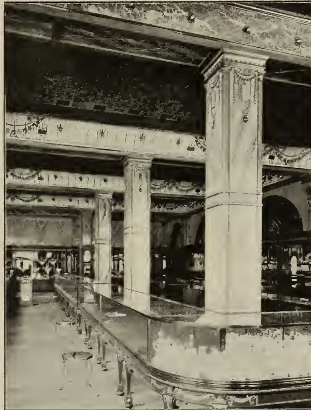
INTERIOR, COLUMBUS MEMORIAL BUILDING, CHICAGO. Column and Ceiling Ornaments in Galvanoplastic, Fire Gilt.
